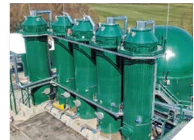
BioPV - Organic waste press water digestion
